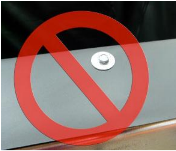
Steel fasteners too close to the water.
