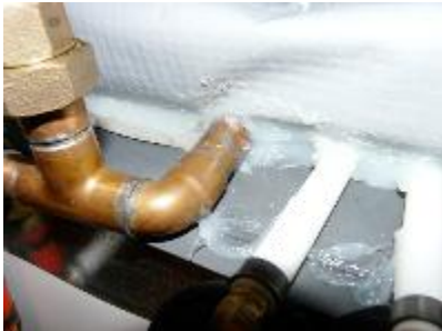
A well-sealed cover and heat exchanger
